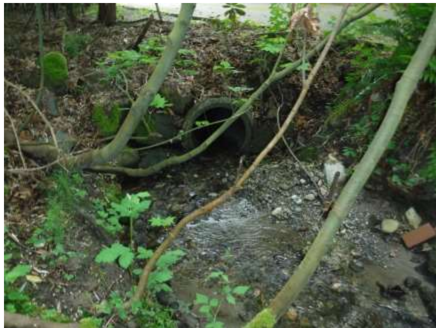
Image 8: Open channel flows inlet this 24" concrete culvert
